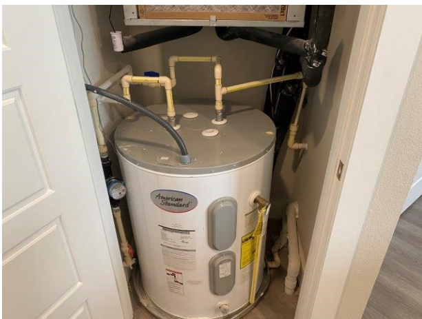
17. Typical apartment electric water heater
