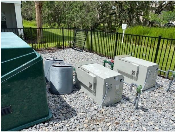
9. Pool heater connected to propane UST
